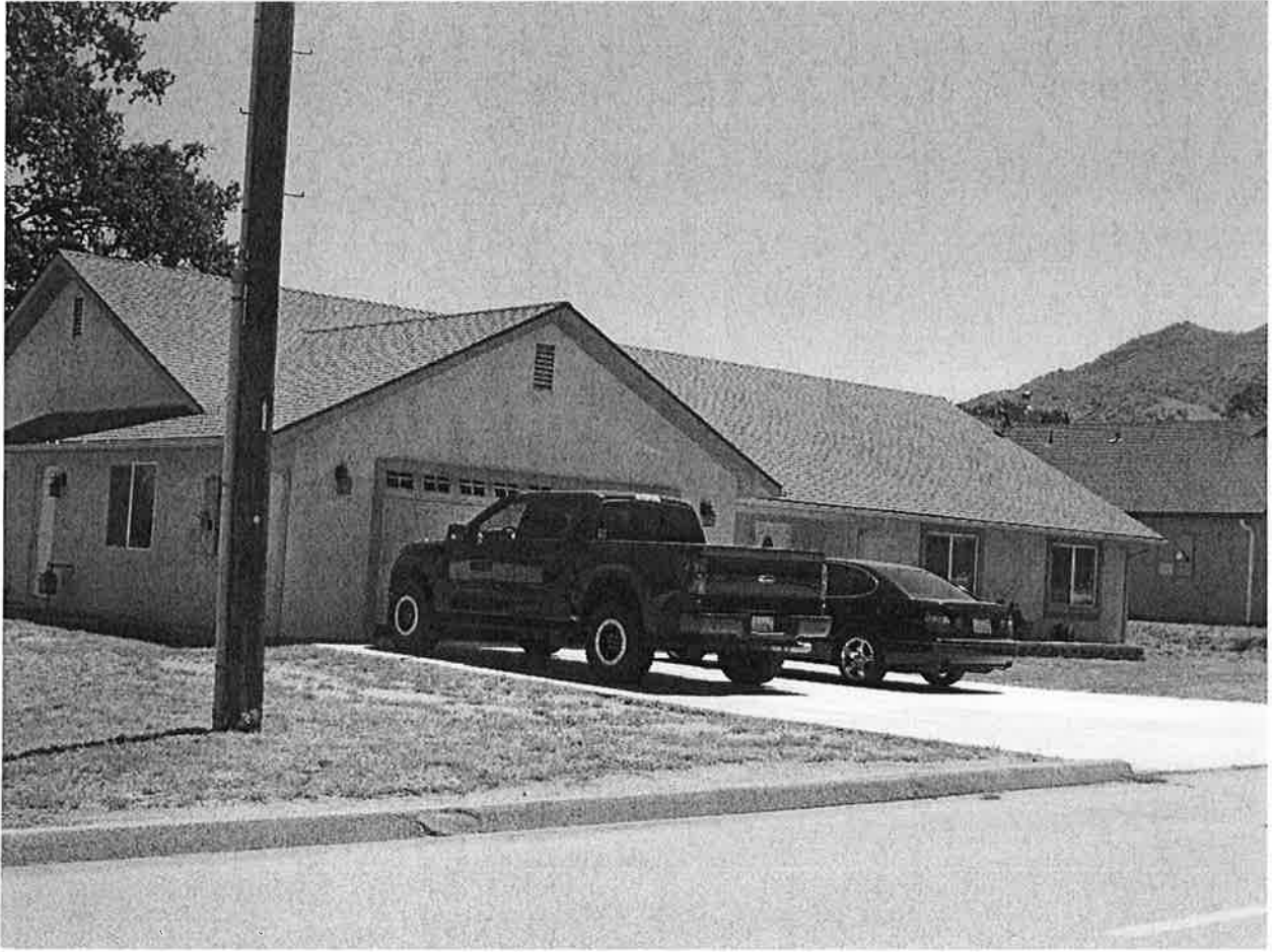
A. Underground power and telephone
